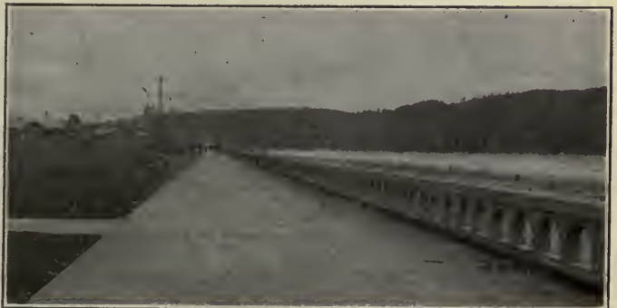
NEW CONCRETE PROMENADE AND SEA-WALL, SEASIDE, ORE.
